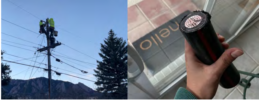
FIG. viii A section of a copper conductor from a distribution line. Donated from linemen who were repairing the lines in my backyard after a blackout caused by high winds. Note the “stranded” nature of the conductor - rather than a solid piece of copper, many smaller, bundled conductors help improve the flexibility of the conductor and can carry more current.
